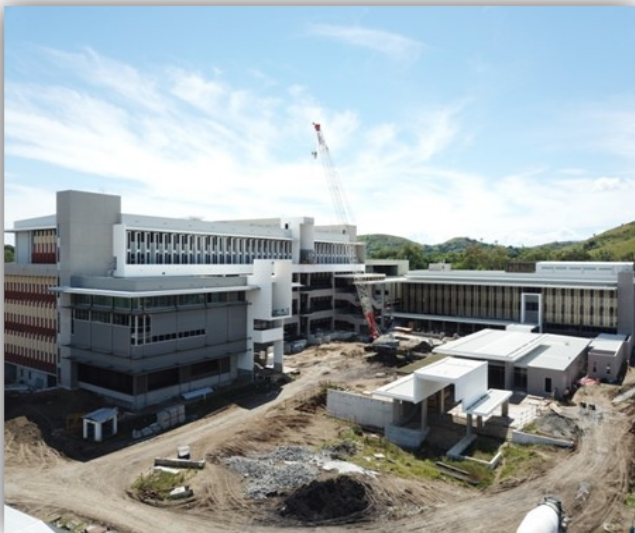
Aerial view from South-West showing construction progress as at 31/12/2020.
