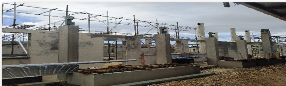
Proposed Bialla Court House – Front Entrance (57% completed)
