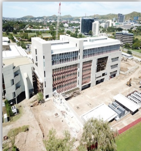
Aerial view from North showing construction progress as at 31/12/2020.
