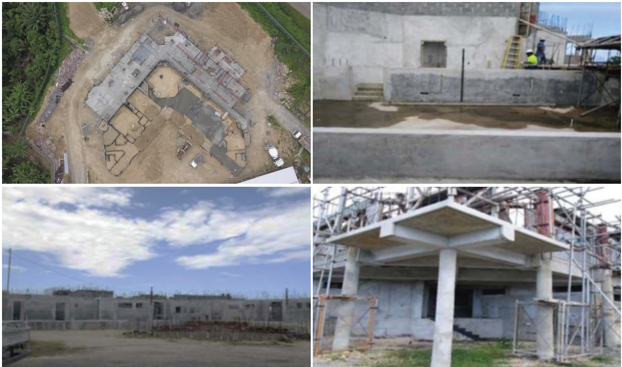
Construction in Progress and work expected to complete in year 2020
