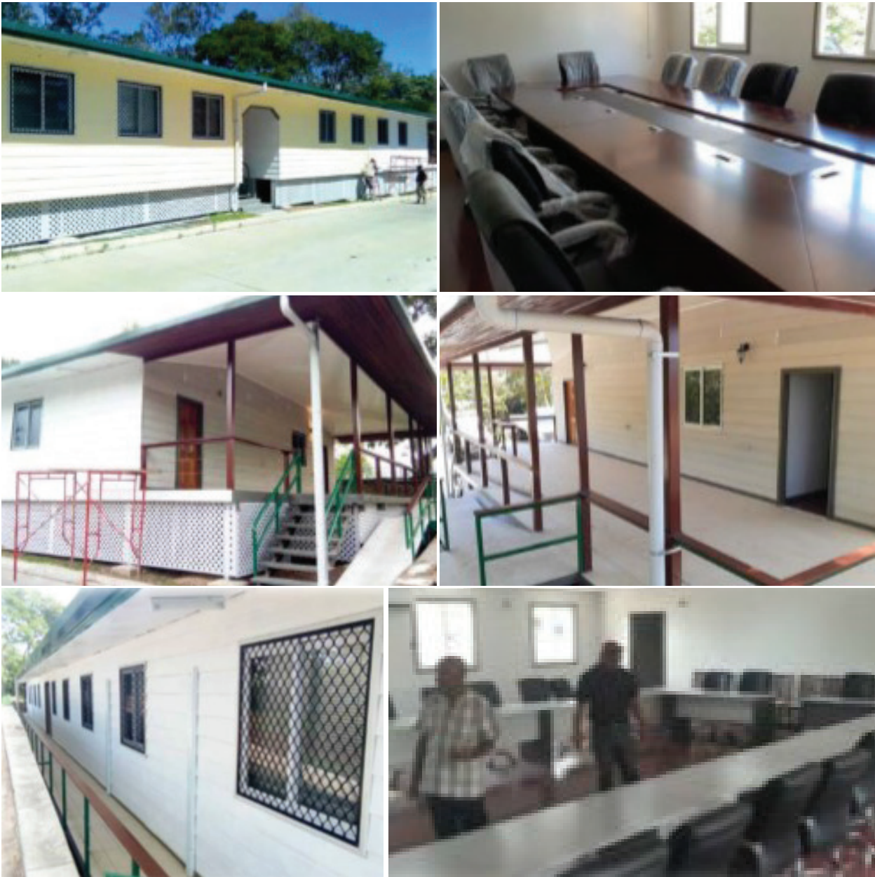
Images of work of the PNGCJE Training Facility almost completed
