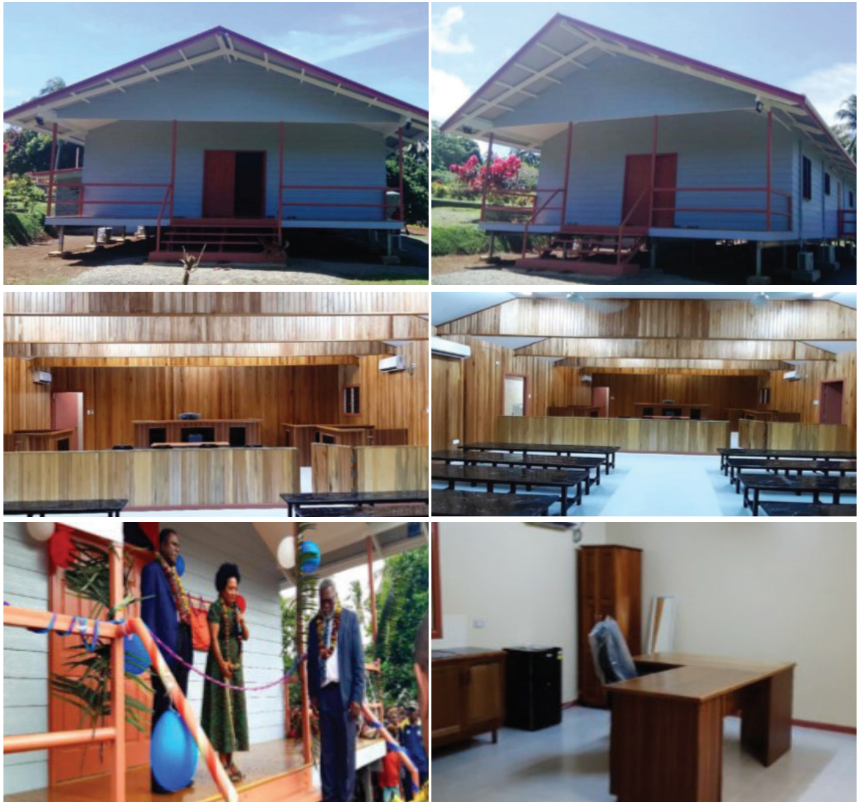
Images of construction completed and the official opening By Justice Ellenas Vitata Batari , CSM MBE
