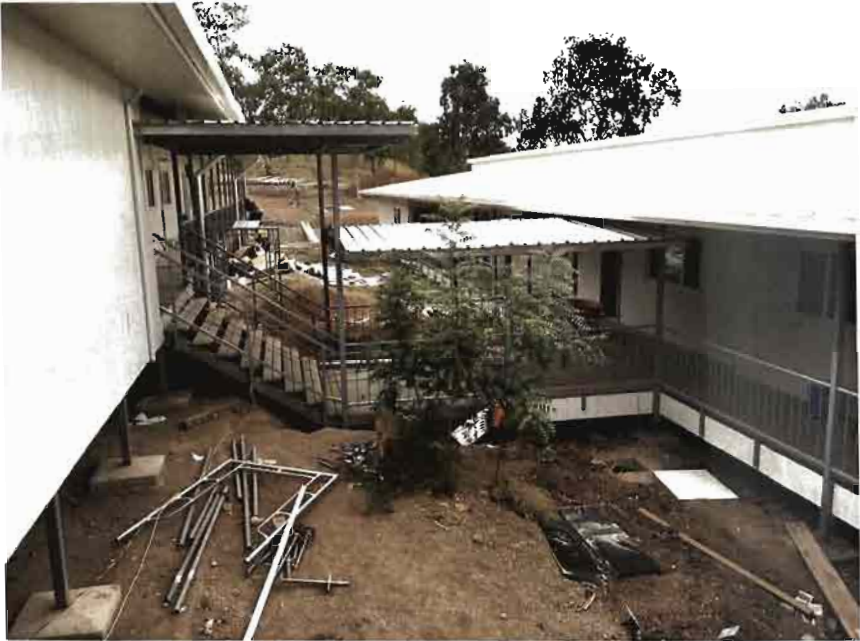
Above the 2 new temporary buildings at Waigani nearing completion
