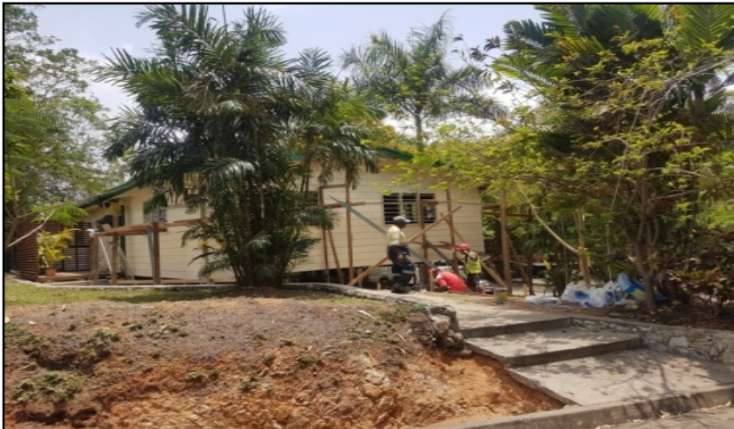
Temporary Office of the PngCJE & PicCJE Executive Director under construction
