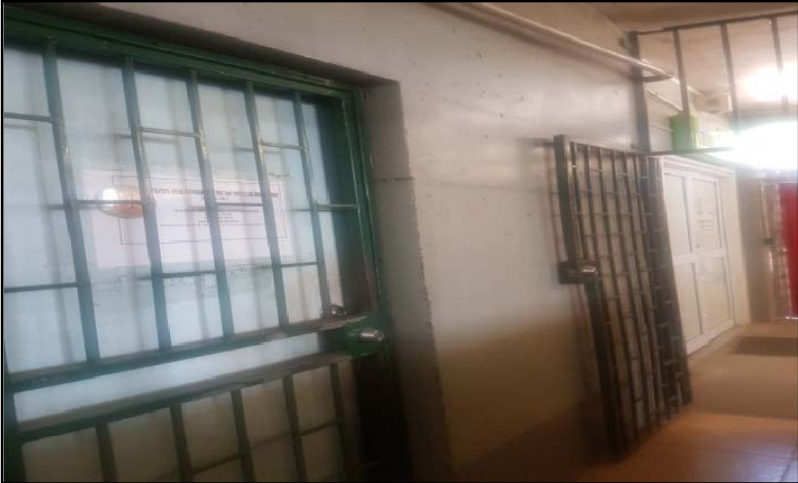
PngCJE Office No. 1 situated in the existing Court building (ground floor)
