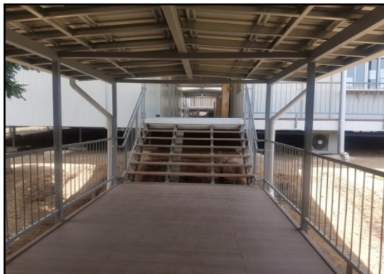
Staff circulation corridors of Admin Wing
